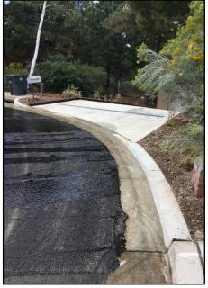
Crews fixed a long-standing drainage issue on a cul-de-sac on North Mesa. During a small rain event sediment was left behind in front of the driveway. If it was a large rain event, the stormwater in the gutter tended to overtop the drive-pad. Crews removed a section of curb and gutter along with lowering the drainage inlet elevation, in order to create a steeper slope in the gutter. This would allow the smaller
