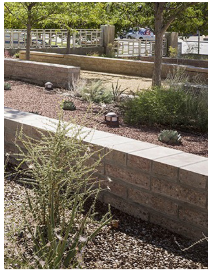
SEAT WALLS - RECYCLED CONCRETE FROM DEMOLISHED SHUFFLE BOARD COURTS
