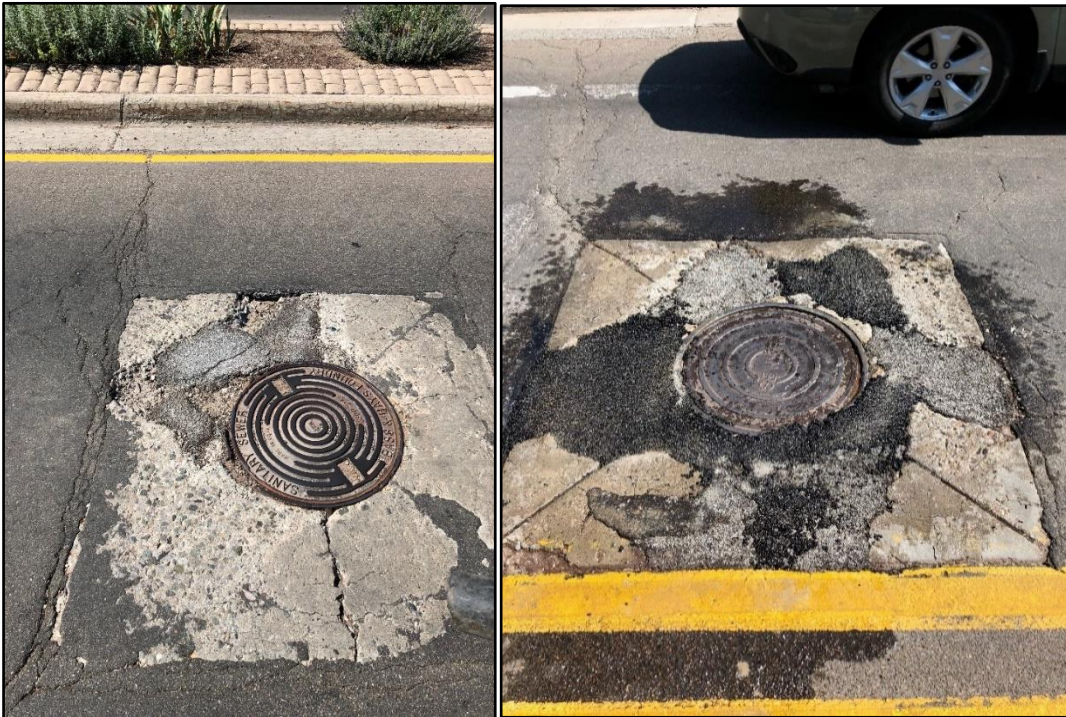
Crews patched around manholes on Canyon Road.
