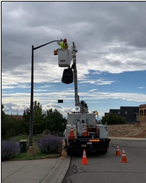
Traffic Electricians replaced an older streetlight fixture with a new LED fixture on Quemazon Street. Crews are monitoring and making adjustments to try and find a balance between lighting the roadway and not interfering with residents' windows, as this streetlight is on a hill.
