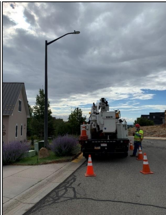
Traffic Electricians replaced an older streetlight fixture with a new LED fixture on Quemazon Street. Crews are monitoring and making adjustments to try and find a balance between lighting the roadway and not interfering with residents' windows, as this streetlight is on a hill.
