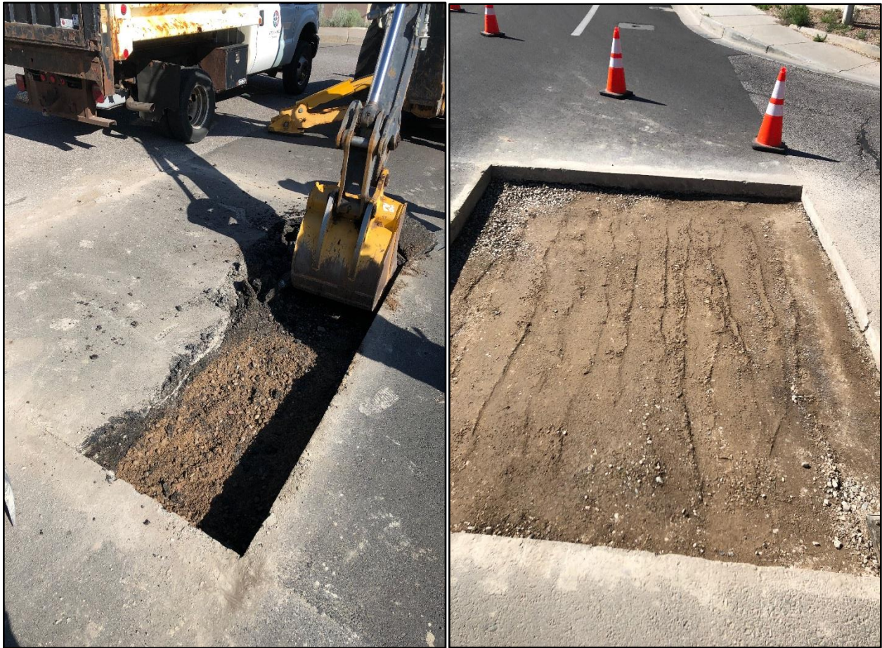
Crews repaired a section of asphalt in the bike lane on Diamond Drive. This area developed a dip as a result of the waterline leak in March.
