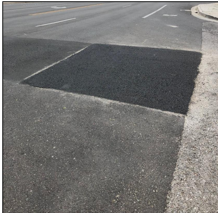
Crews repaired a section of asphalt in the bike lane on Diamond Drive. This area developed a dip as a result of the waterline leak in March.
