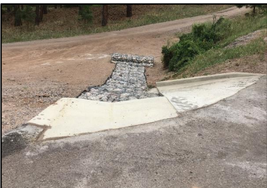
Crews built a rip-rap drainage outlet at the bus turn around on Range Rd.
