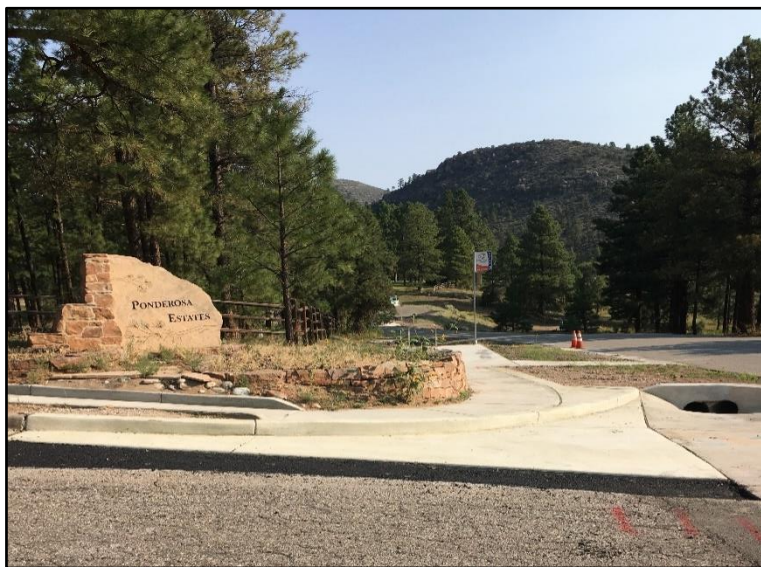
Crews put a radius on curb and gutter for better drainage and added 1 foot of sidewalk for ADA compliance on Range Rd. and Aspen Dr.
