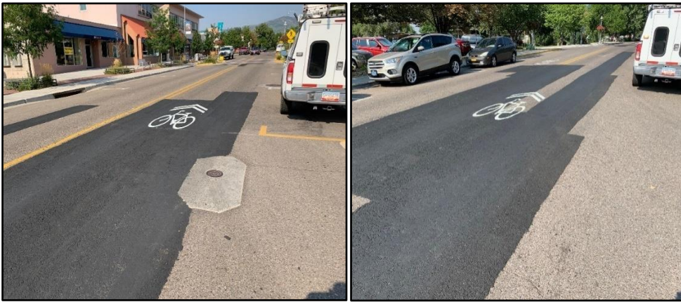
Crews came in at 5:00 AM to replace the sharrows (pavement markings that indicate bicycle and vehicle shared lanes) on Central before the morning rush. Crews also restriped the double yellow lane lines, after the pavement preservation project was completed.
