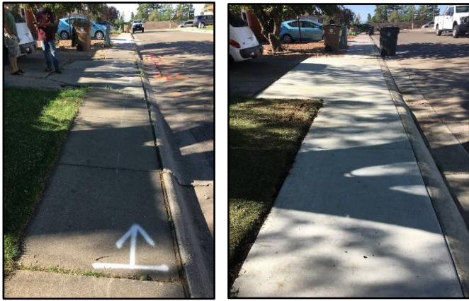
Crews repaired sidewalk, drive pad, and curb and gutter on Nambe Loop.
