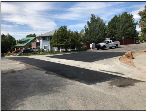
Crews repaired sections of asphalt on Estates Drive.
