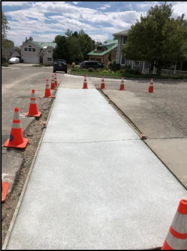
Crews installed a valley gutter on Estates Drive.
