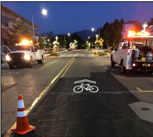
Crews installed several pavement markings on Central. The work was completed in the early morning hours to avoid traffic delays for motorists.
