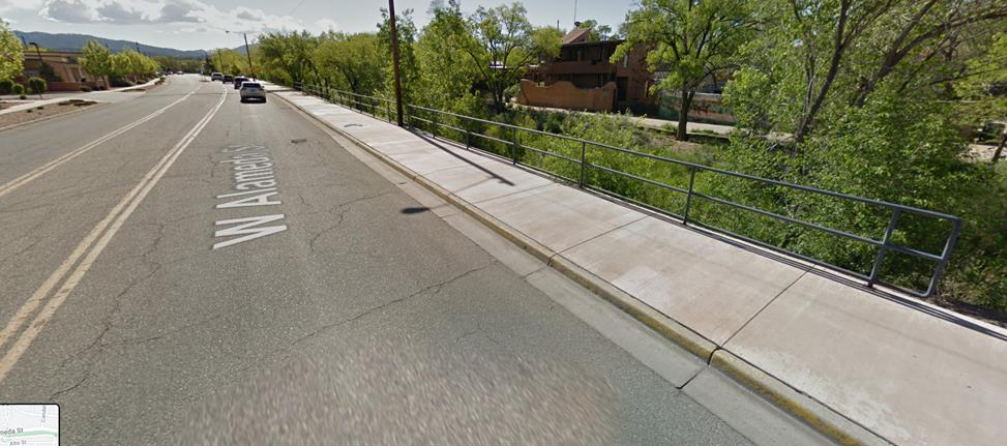
Raised Concrete Path
