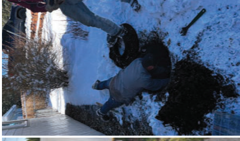
Gas Water Sewer ~Water Meter Change-out~
