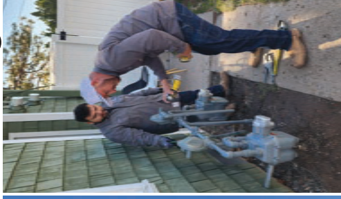
Gas Water Sewer ~Gas Meter Check~
