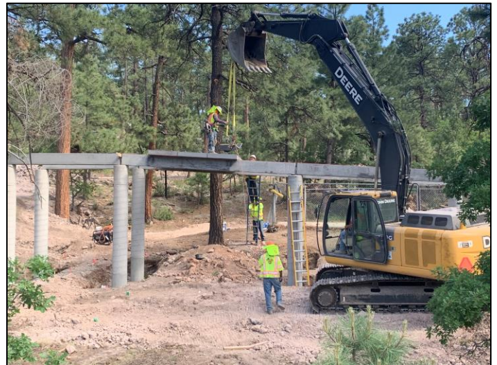
Urban Trail –installation of boardwalk
