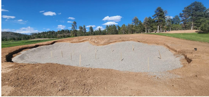
New Bunker on Hole #5
