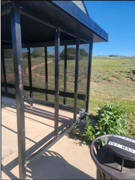
Facilities repaired a bus shelter on North Mesa
