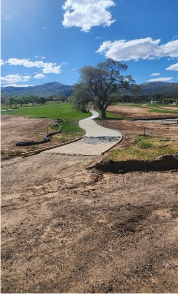
New Concrete Golf Cart Path
