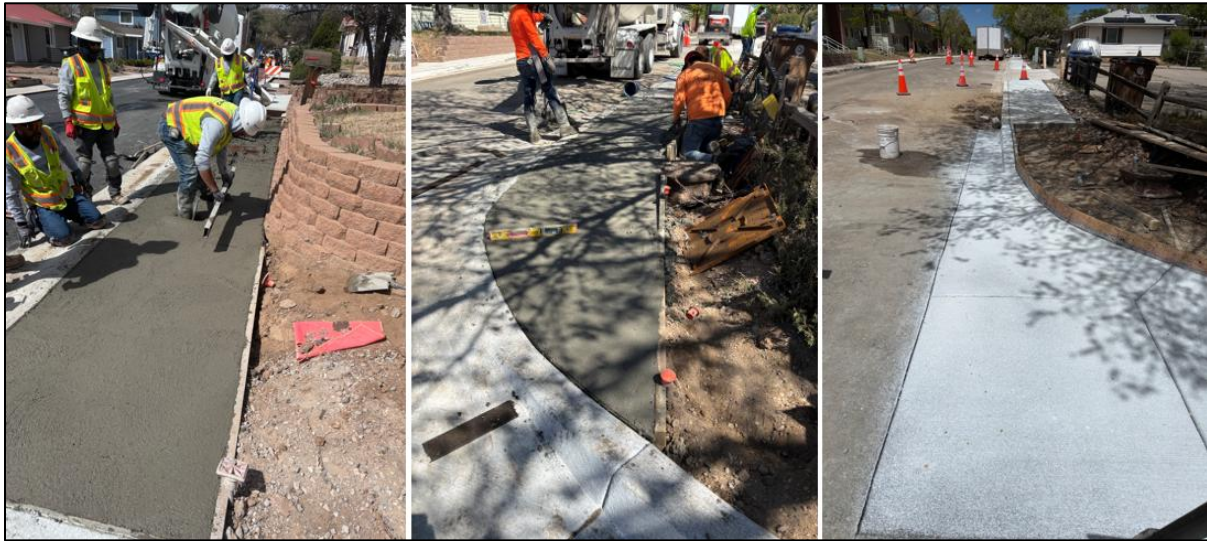
ADA ramps, curb and gutter and sidewalks along 9th Street.
