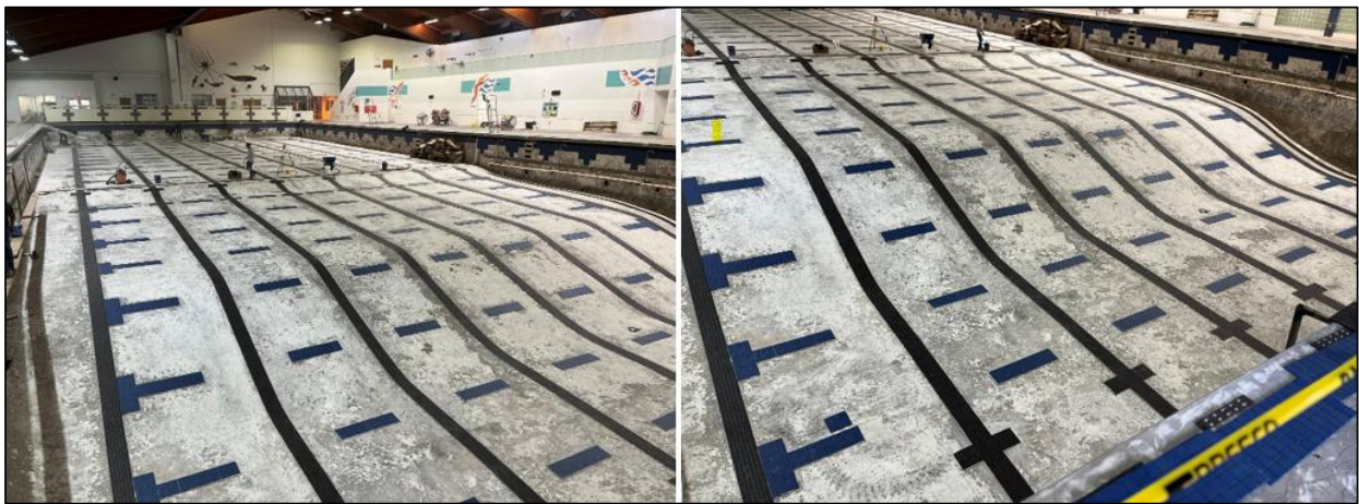
Swim Lane Tile Installation
