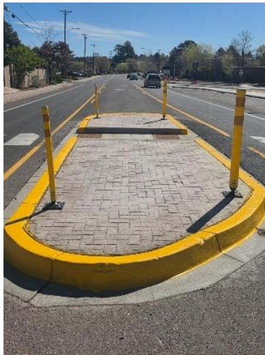
Curb and Island Painting Countywide
