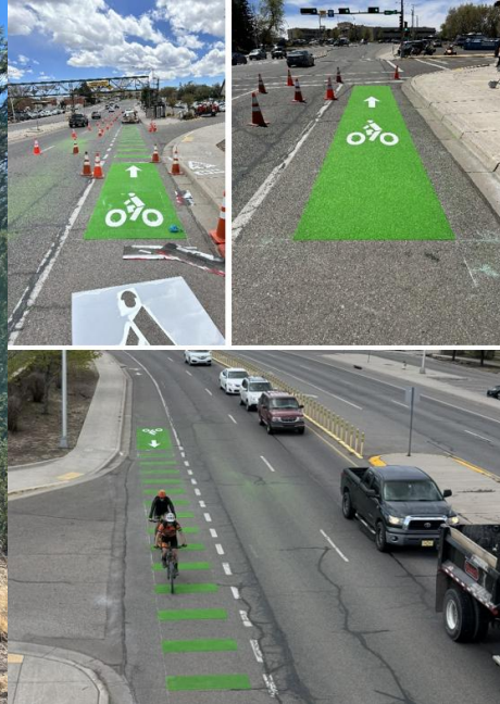
Green Bike Lane Installation
