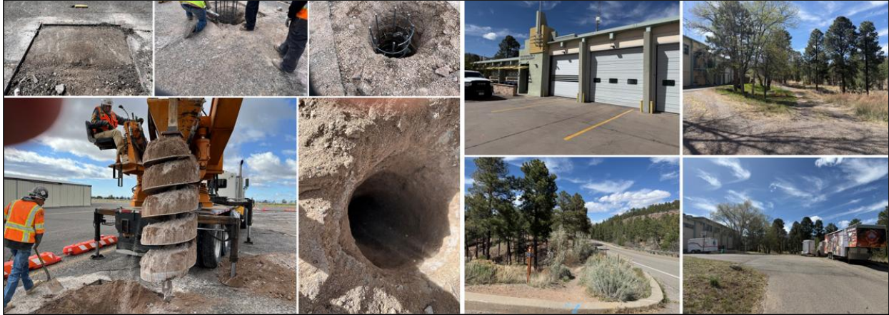
T-Hanger Concrete Pier Drilling
