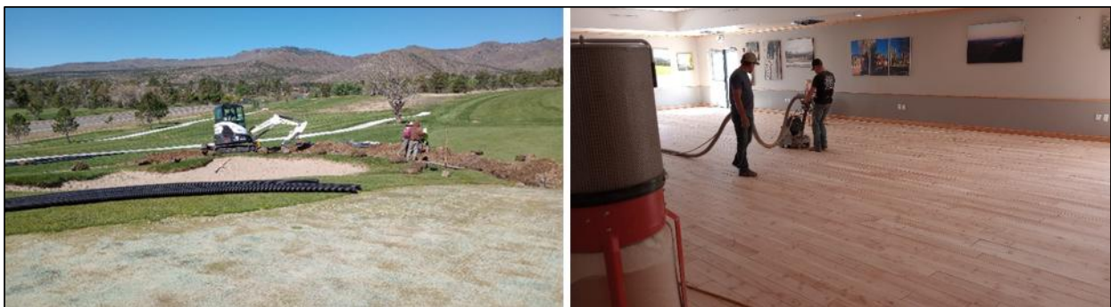
Drainage correction at Golf Course tees and greens. Contractors re-finishing the Community Room wood floors at the Golf Course Clubhouse.
