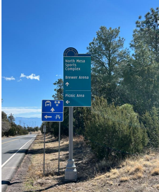
Wayfinding Sign Installation
