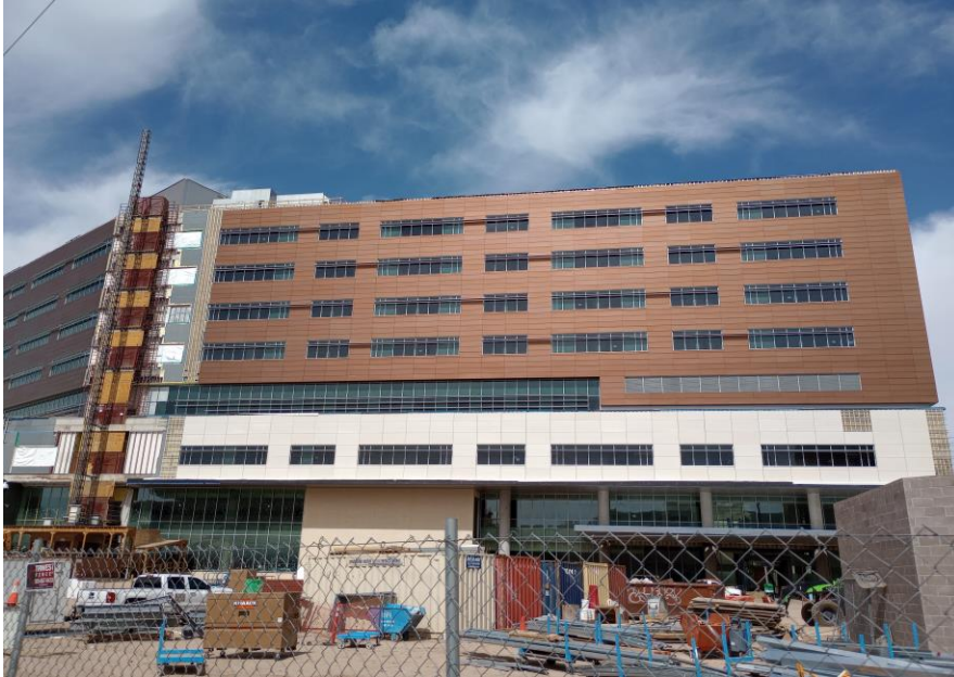
B - MPL Library Siding and Crack Seal Project
