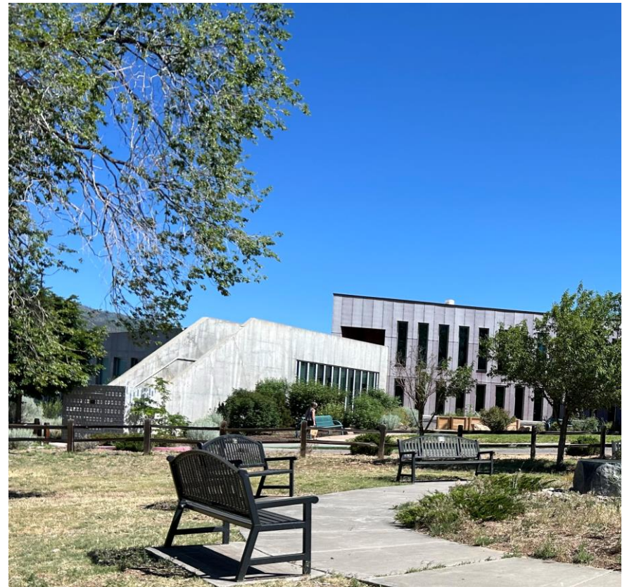
Current Siding Condition 2024
