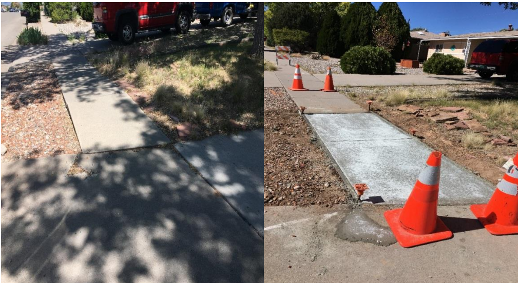
Crews replaced a section of buckled sidewalk at 316 Meadow.
