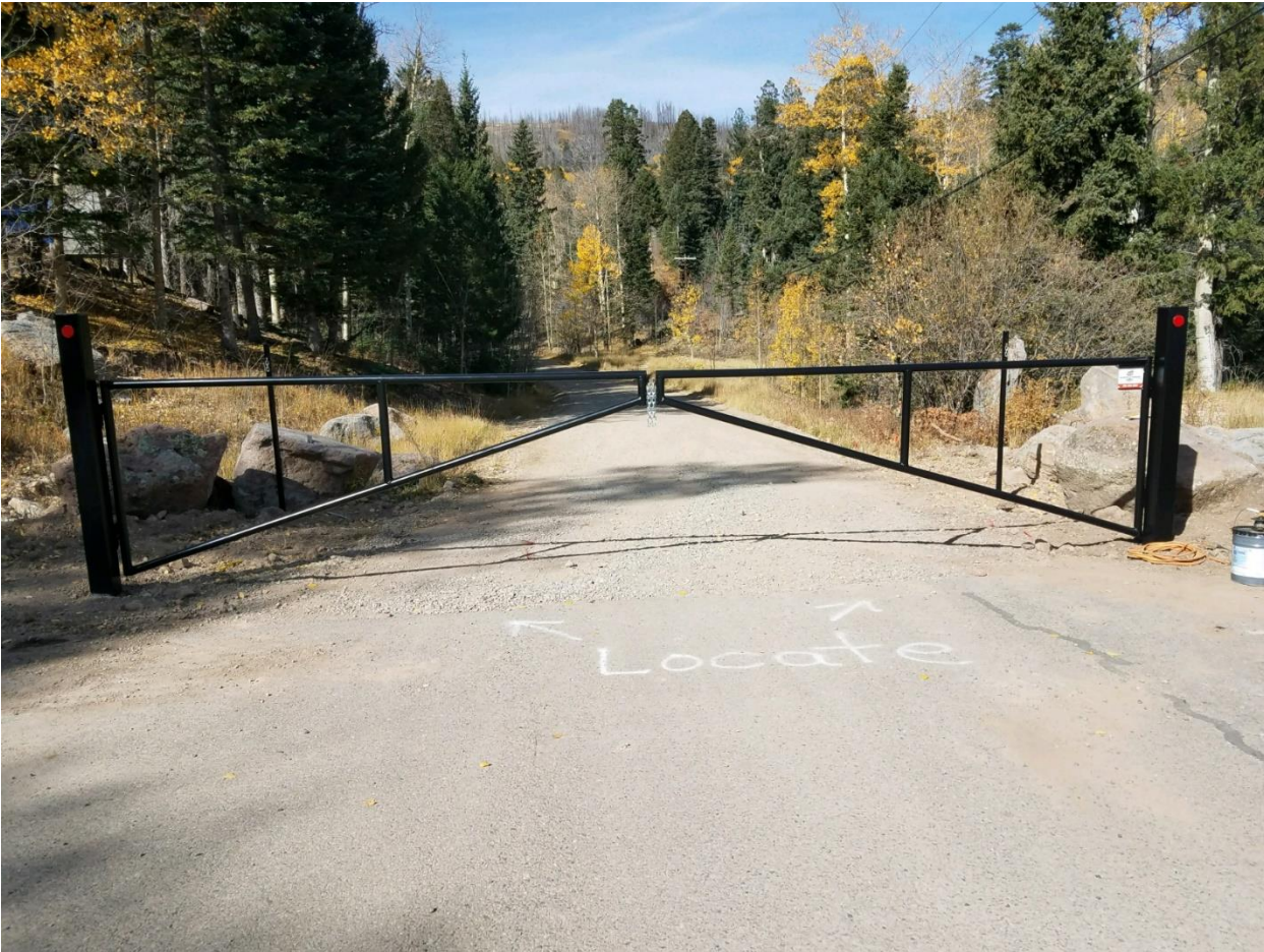
A gate was recently installed by a County contractor on Camp May Road near the base of the ski area to avoid the placement of boulders in the roadway during the winter months.
