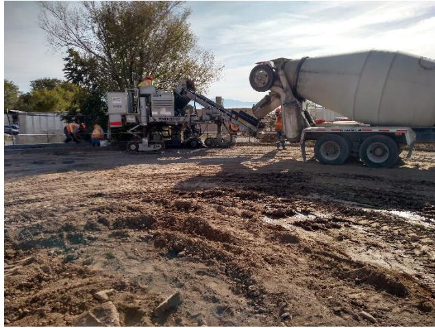
Curb and Gutter Machine
