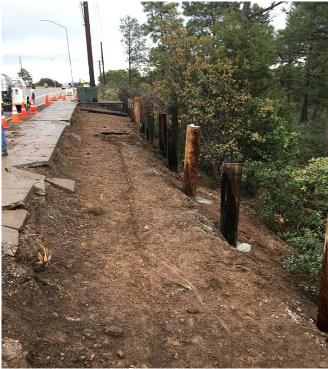
Crews removed a large section of sidewalk, and reinforced a new section of sidewalk with a retaining wall along San Ildefonso Road.
