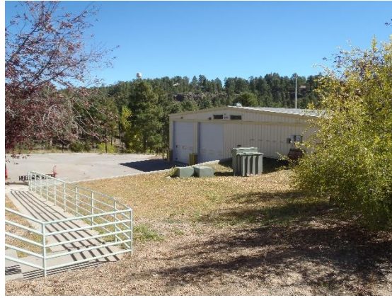
Temp Trailers Removed, Doors Painted
