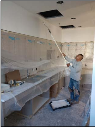
The renovation of the DPU Standby Area is almost complete. During the month of April, contractors worked on texturing and painting walls and ceilings, tiling floors and walls in bathrooms, installing flooring and carpets, installing casework and appliances.
