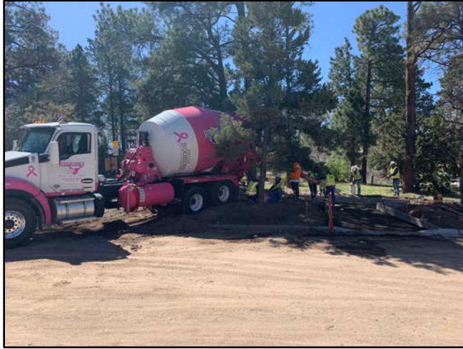
Concrete work on Rose Street
