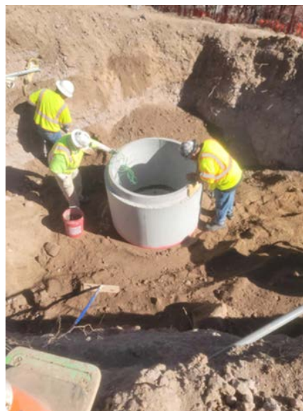
Fuel Farm Project at the Airport
