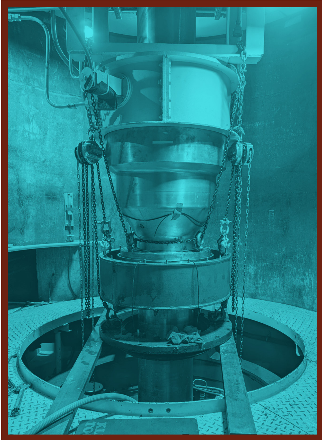
El Vado's operators completed the turbine shaft seal replacement.
