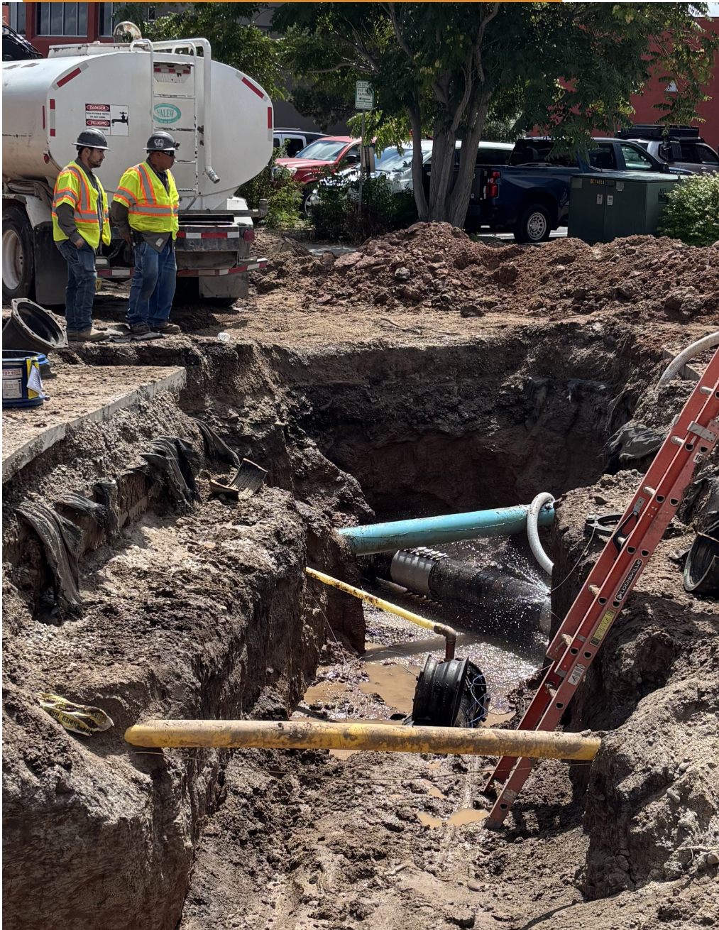
GWS monitored the replacement of a large water transmission line on 15th Street near Central Park Square during the Public Works Department's portion of the Bathtub Row Reconstruction Project.
