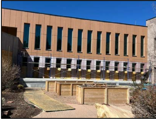
Siding install in progress
