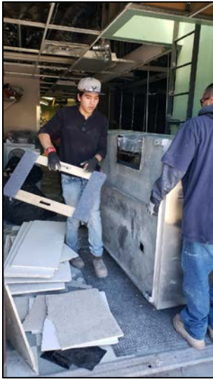
Kitchen renovations at Betty Ehart Senior Center
