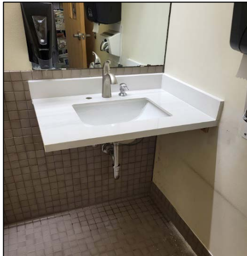
Sink replacement at Mesa Public Library
