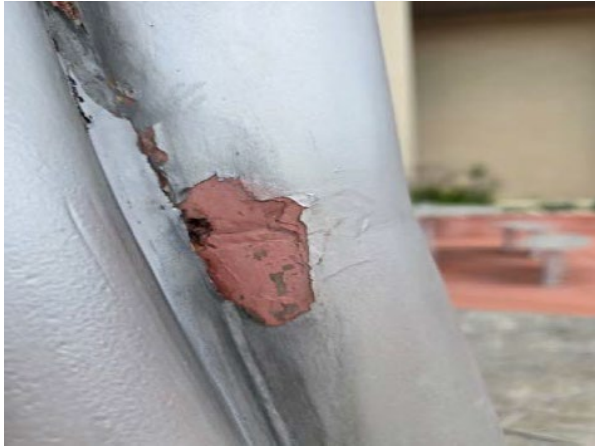
Detail: Area of failed paint pulled back to a stable point prior to painting
