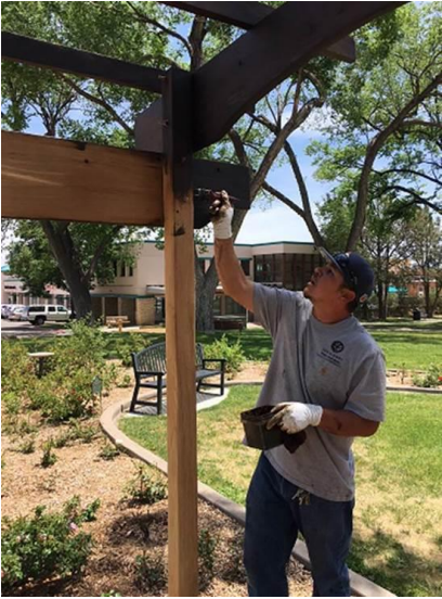
Painting continues at Overlook Concession Stand. 90% complete:
