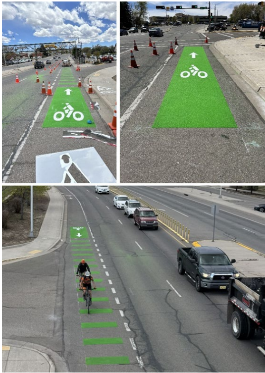
Green Bike Lane Installation
