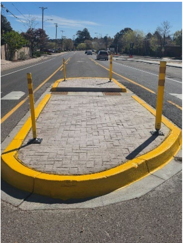
Curb and Island Painting Countywide
