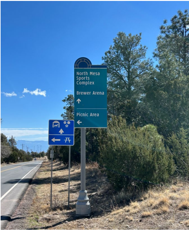
Wayfinding Sign Installation
