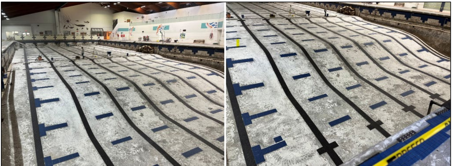
Swim Lane Tile Installation
