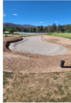
New Bunker on #6
