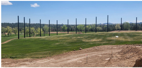
New Practice Range pole (1 st 2 sections)
