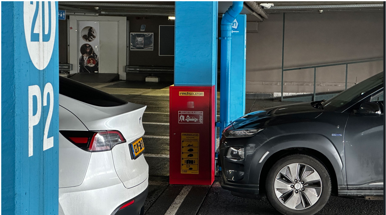
Figure 4-5: Fire isolator cabinet
