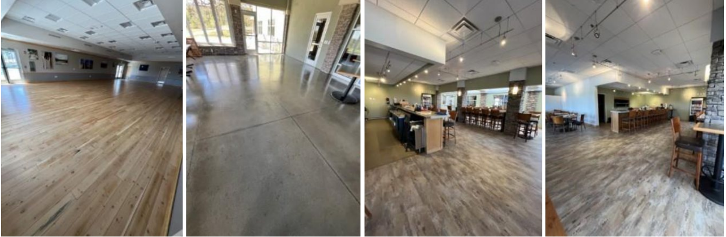
Golf Course Community Room, Patio, Dining Room Re-finish and Granite Countertops
