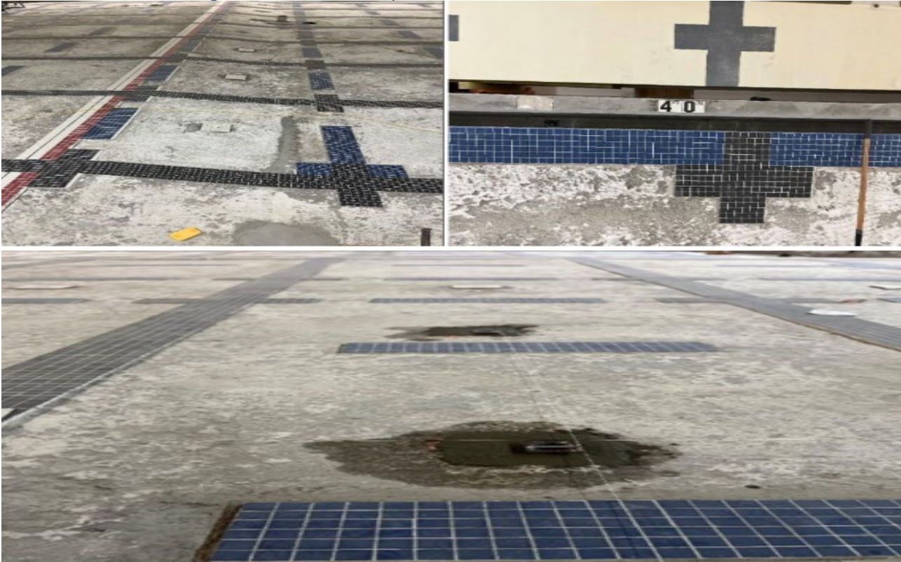
New Tile Installation Along Swim Lanes and Depth Indicators as Well as New Under Water Anchor Installed.
