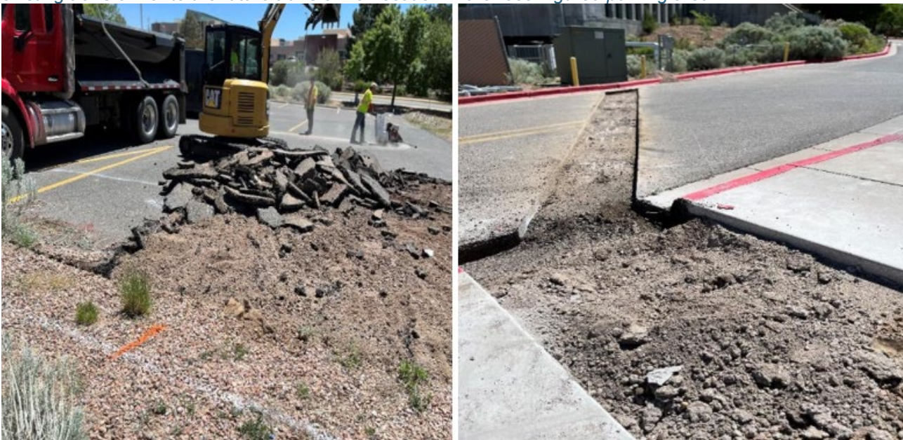
Mesa Public Library EV charging station project: crews trench and remove asphalt to run new electrical conduit from the existing transformer to the future transformer location in the reconfigured parking area.
