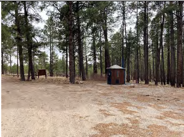
Parking area, turnaround and restrooms
