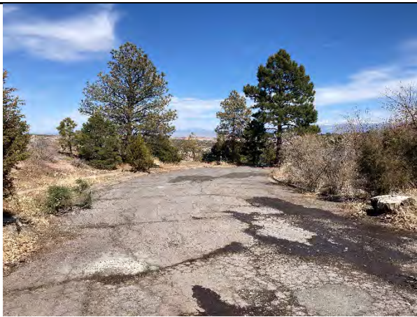
Barranca Rd walkup and undefined parking area
