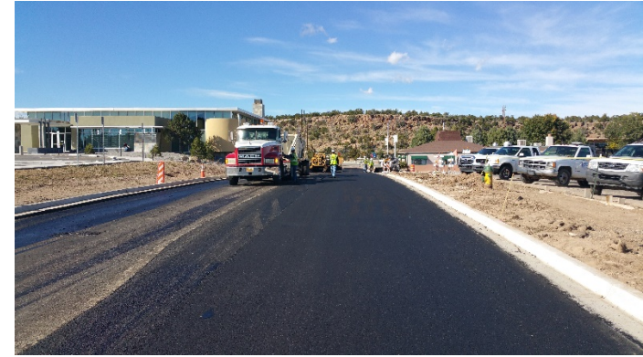
Paving and striping.
