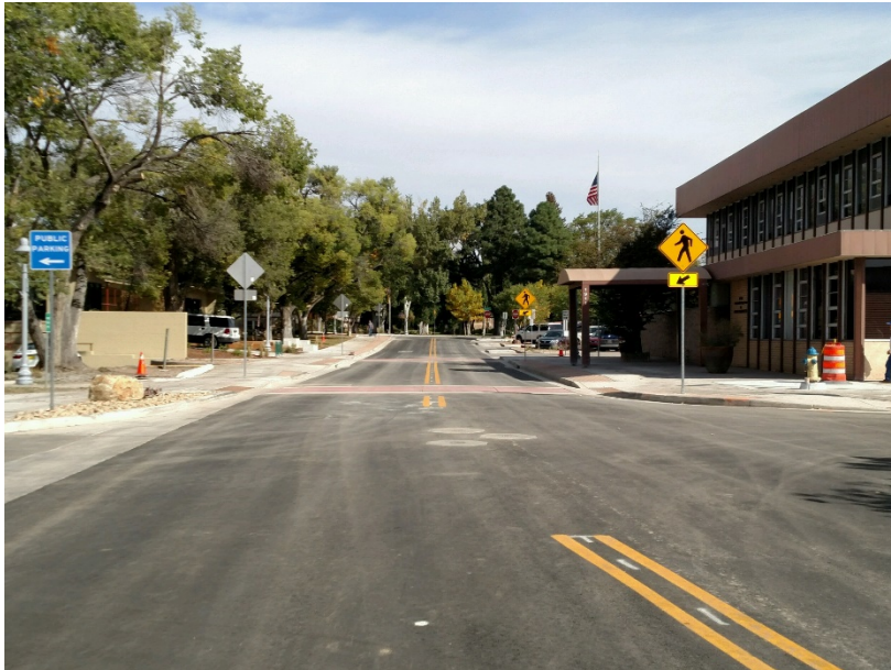
20th Street Improvements
