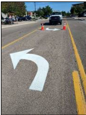
Roadway Striping on Central
