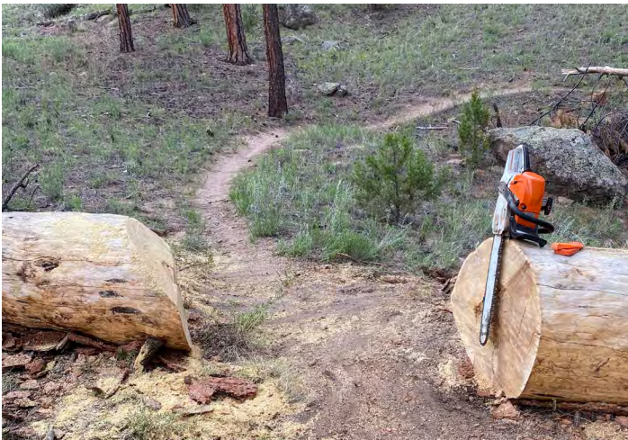
Widen trail tread where necessary.
