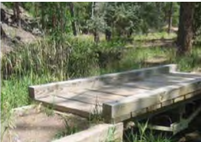
Monitor bridge condition.
