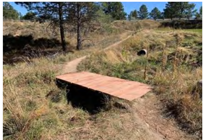
Monitor condition of bridges.
