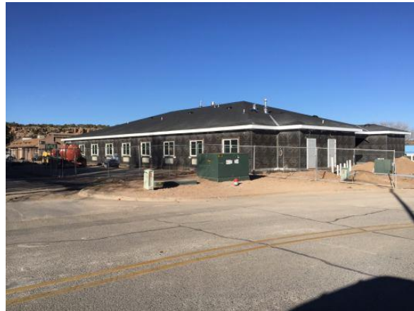
Construction of Bee Hive Homes (White Rock)
