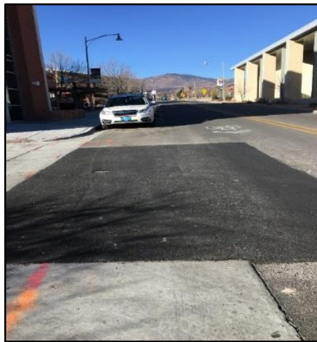
Crews assisted Utilities and re-patched a street/pavement cut at 999 Central
