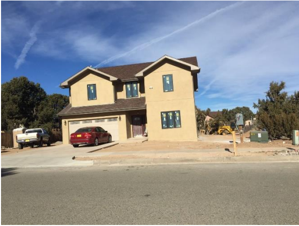
New Residence on Grand Canyon (WR)
