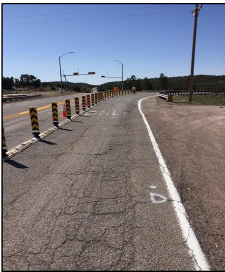
Crews replaced vertical panels in the center median at Trinity & 39 th Street and on State Road 4.
