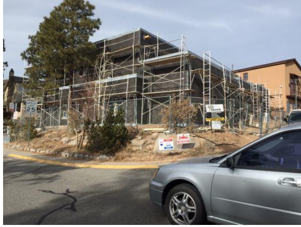
Construction of Four Town Houses in Quemazon (LA)
