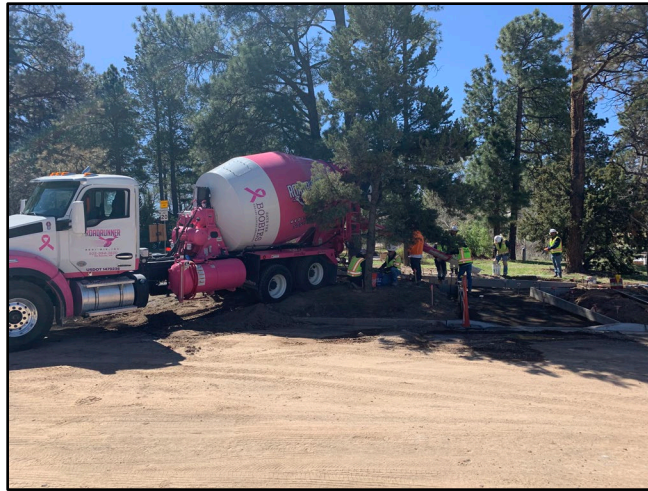
Concrete work on Rose Street
