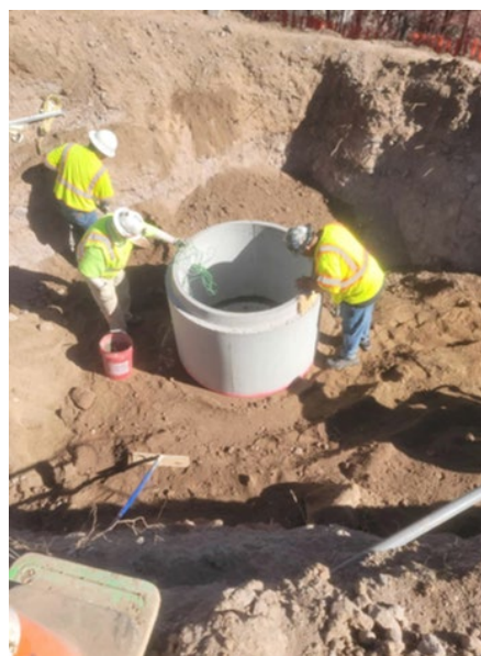
Fuel Farm Project at the Airport
