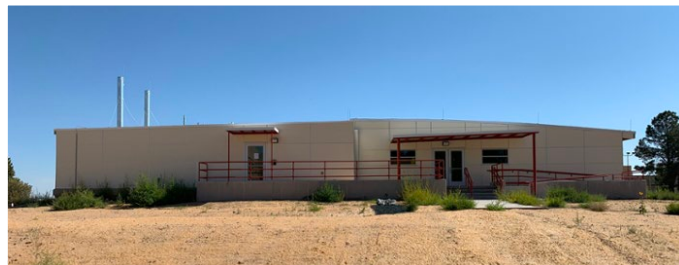
Bio lab & office facility: complete
