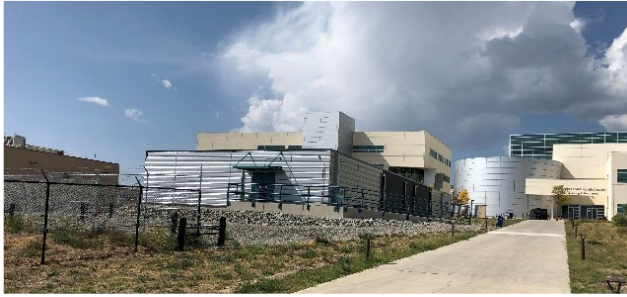
Secured office facility: complete
