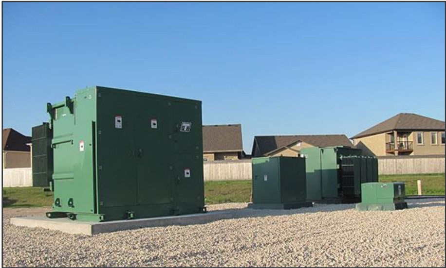
Figure 4-27: Modular Substation Example from Manitoba Hydro
