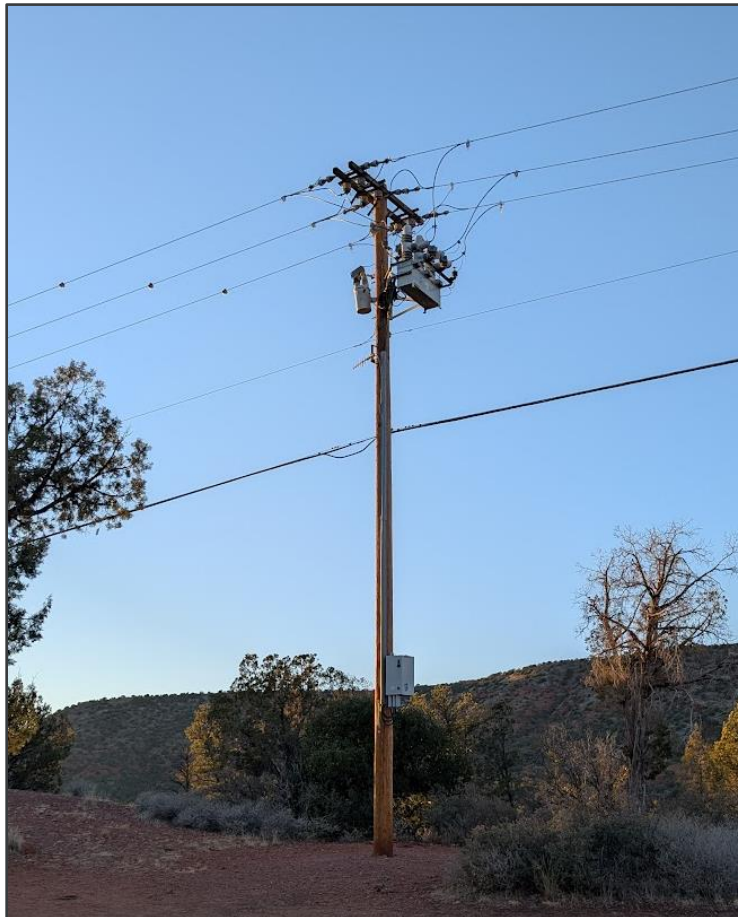
Figure 4-25: Distribution Line Recloser
