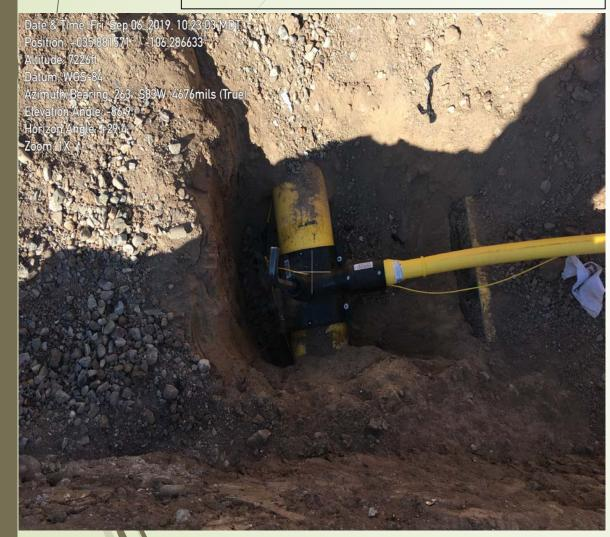
Temporary Pressure Testing Pipeline Run to Pressure Testing Equipment.
