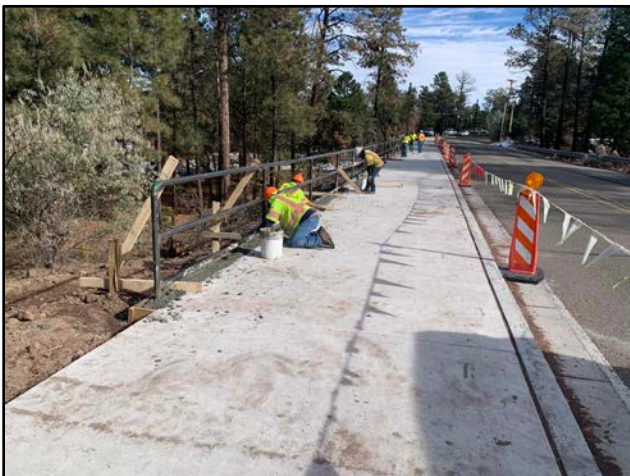
Urban Trail safety railing installation continues.
