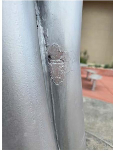
*Detail: Area of failed paint pulled back to a stable point and then painted.*
