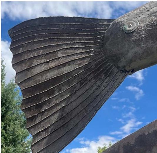
*Detail with failing coating before treatment.*
