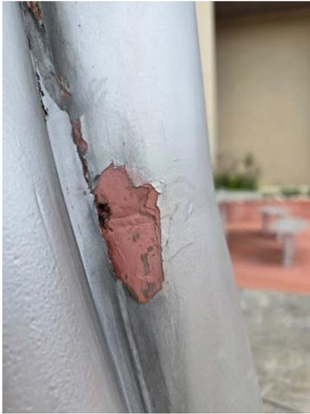
*Detail: Area of failed paint pulled back to a stable point prio to painting*
