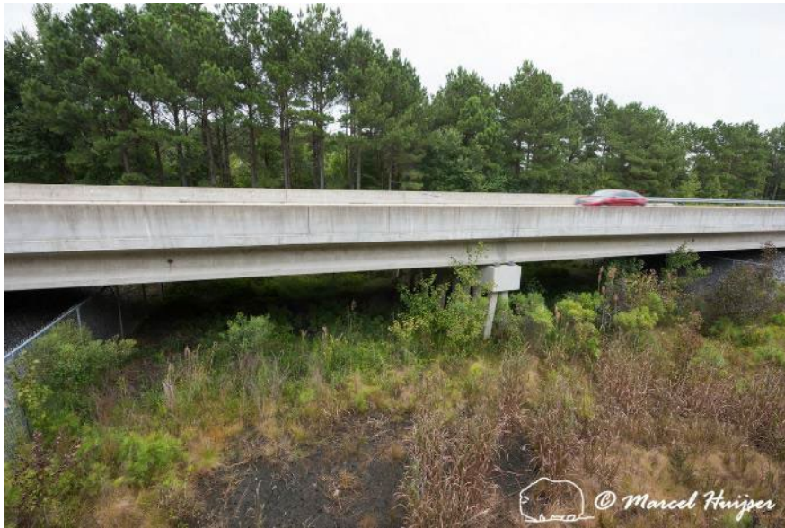
Figure 79. Wildlife underpass and fence with grasses, shrubs, and trees in the median and also some under the bridges, US Hwy 64, near Roper, North Carolina, USA.
