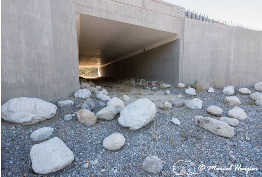
Figure 91. Boulders provide cover to small animal species and block access to unauthorized vehicles at wildlife underpass, US Hwy 95, Chilco, Idaho, USA.
