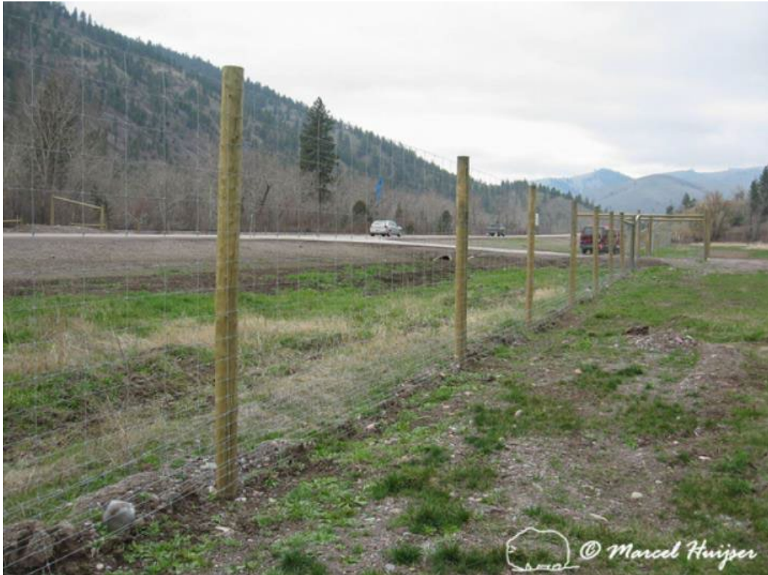
Figure 7. Typical large ungulate fence in North America, 8 ft tall, wooden posts and mesh-wire fence material, US Hwy 93 North, Montana, USA. Note that there is a dig barrier attached to the main fence material (e.g. for canids).
