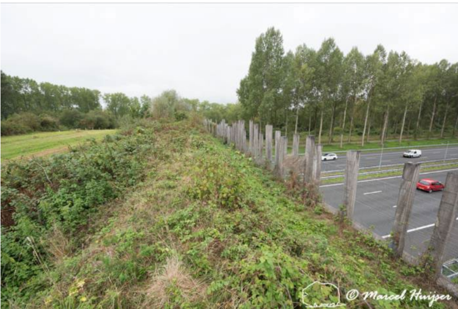
Figure 18. Berm on wildlife overpass "Groene Woud" across A2 motorway, The Netherlands. The berm with rootwads and shrubs provides cover on either side and reduces visual and noise disturbance barrier combined with large mammal fence on an overpass, The Netherlands.
