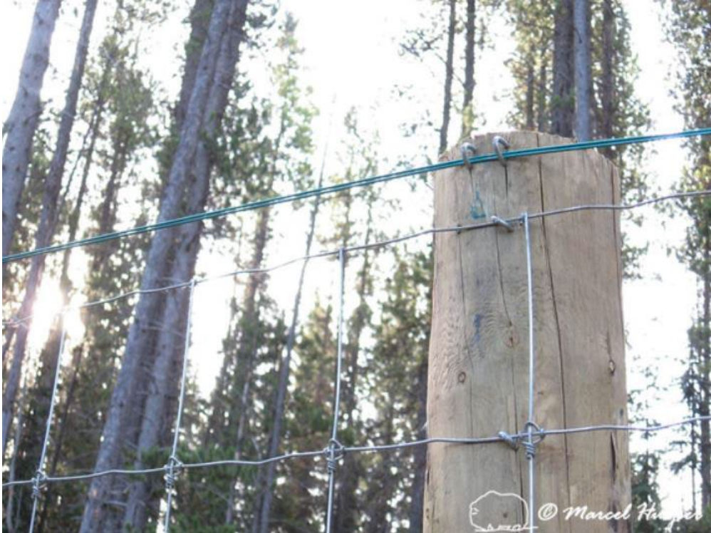
Figure 11. Wildlife fence with high-tensile top wire to reduce damage from falling trees, Trans-Canada Highway, Banff National Park, Alberta, Canada.
