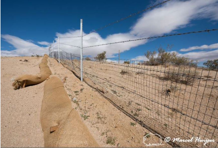
Figure 67. Fence to keep desert tortoise ( Gopherus agassizii ) off the highway, California, USA.
