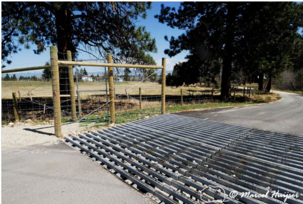
Figure 33. Wildlife guard at an access road to US Hwy 93S, near Victor, Montana, USA. This type of wildlife guard is less suited for pedestrians and cyclists.
