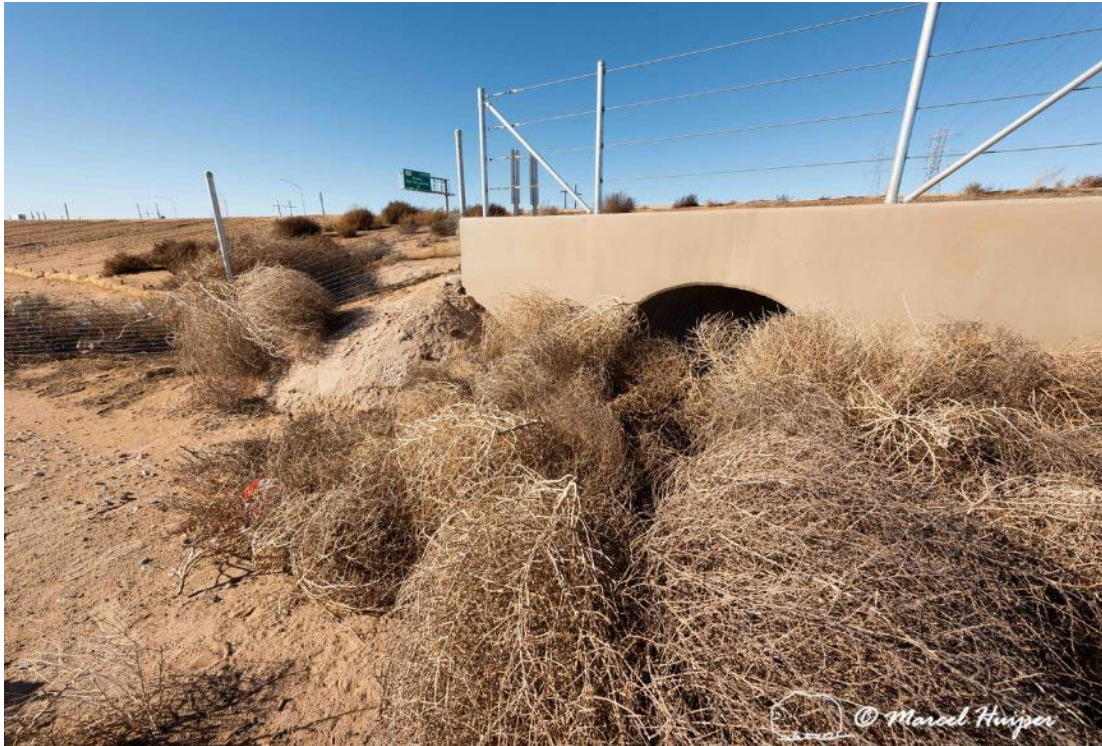
Figure 95. Tumbleweed blocks culverts, primarily for hydrology, but also for Mojave desert tortoise ( Gopherus agassizii ), Hwy 58 near Kramer Jct, California, USA.
