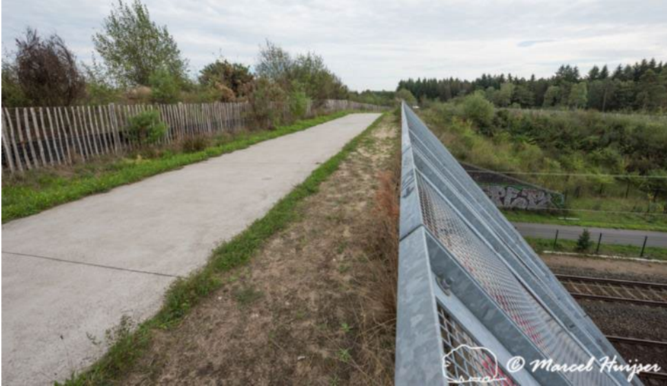
Figure 22. Hiking and biking trail combined with wildlife overpass across railroad tracks, Soest, The Netherlands. The “wildlife area” on the overpass is further to the left, separated from the trail by a berm and shrubs and trees.
