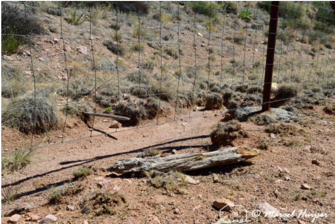
Figure 51. Wildlife fence does not connect to the ground, Arizona, USA. Animals may be able to crawl under the fence.
