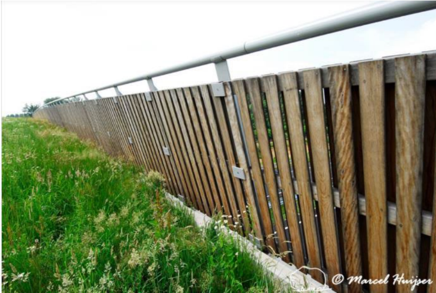
Figure 17. Visual barrier combined with large mammal fence on an overpass, The Netherlands.
