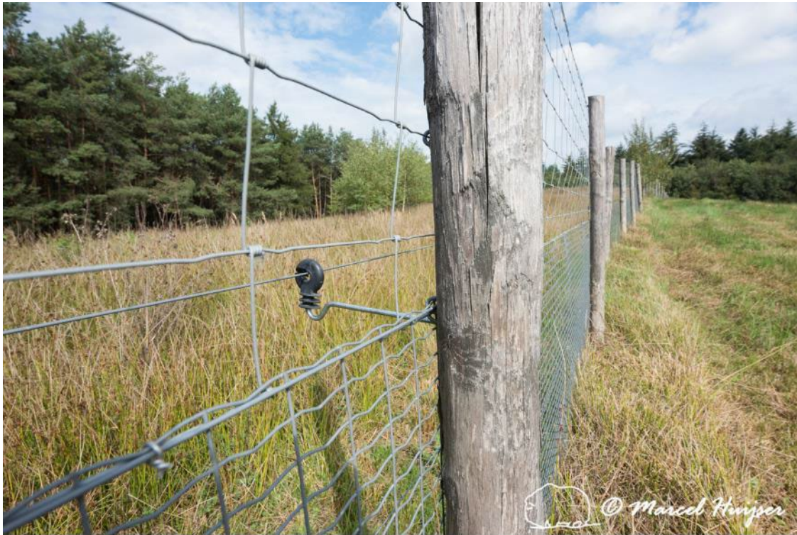
Figure 76. Wildlife fence along A28 motorway, near Spier, Drenthe, The Netherlands. The fence is a barrier for medium and large mammal species. The electrified wire is an additional barrier to keep animals from climbing the fence.
