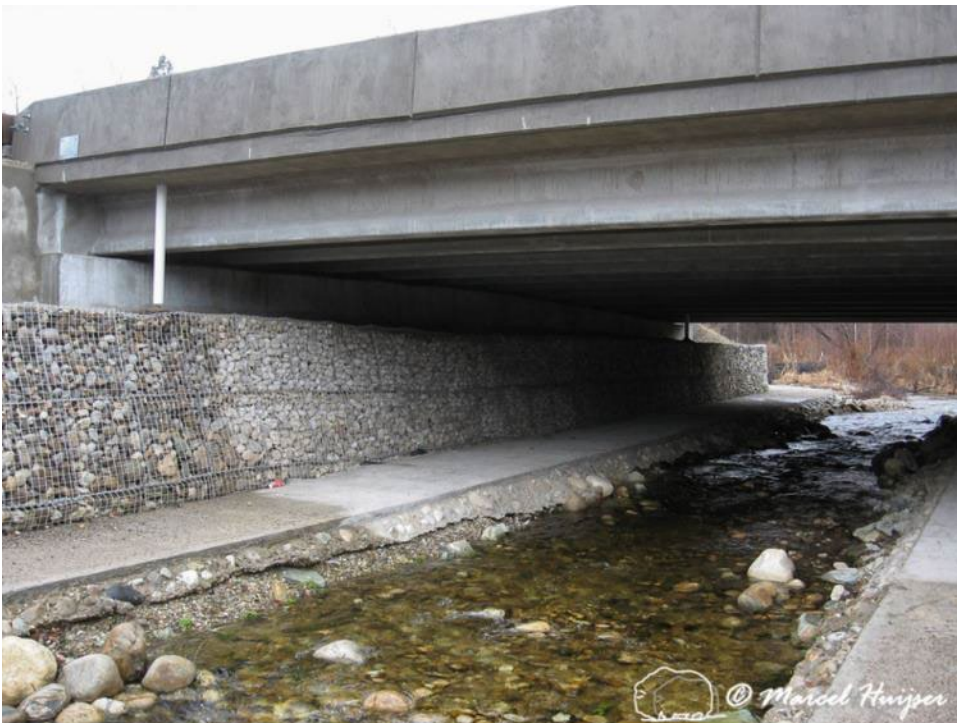
Figure 23. Pathway for large mammals in an underpass (bridge) primarily designed for water (stream), US Hwy 93 S, Bitterroot Valley, Montana, USA.
