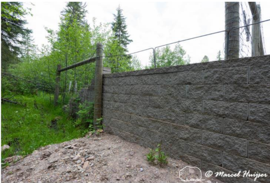
Figure 46. Wildlife jump-out along US Hwy 93, Flathead Indian Reservation, Montana, USA. Jump out is 5 ft tall with rebar on top.
