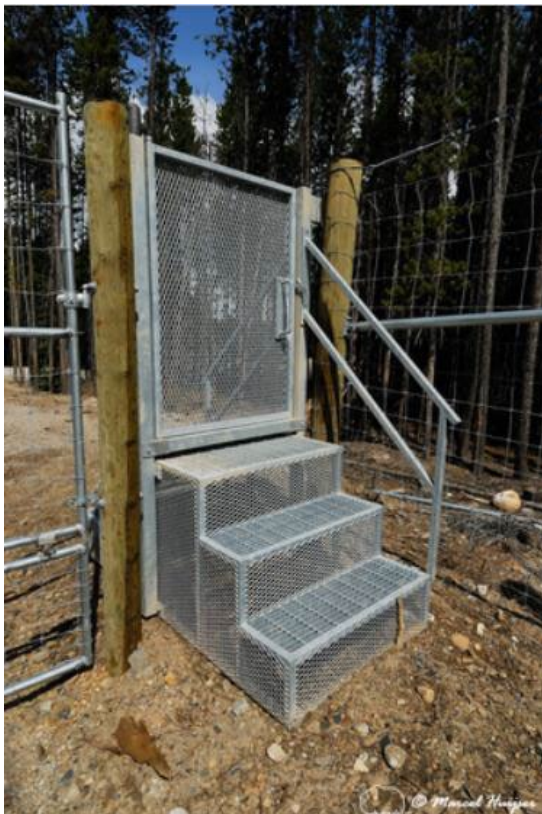
Figure 43. Pedestrian gate with steps (for high snow accumulation) at a wildlife fence, Alberta, Canada.
