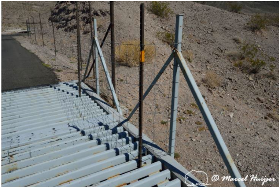
Figure 35. Blocked concrete edge at side of wildlife guard at access road US Hwy 93, Arizona, USA. Some wildlife species will walk on the narrow concrete edge of the wildlife guard to access the fenced road corridor. The concrete edge is part of a wall for the pit under the metal bars. Here the edge is made inaccessible to large mammals through an extra piece of wildlife fence.
