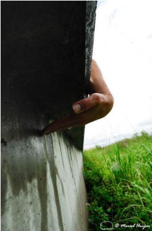
Figure 72. Barrier wall integrated into the roadbed with overhang for reptiles, amphibians and small mammals, U.S. 441, Paynes Prairie Ecopassage, south of Gainesville, Florida, USA.
