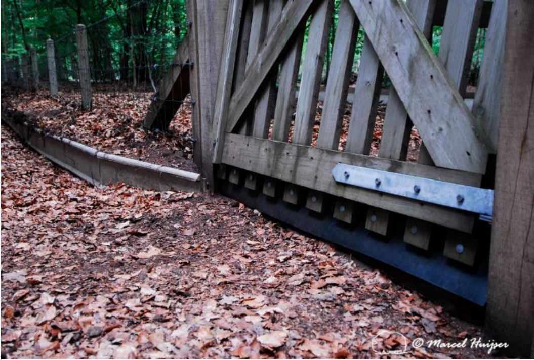
Figure 103. A gate for pedestrians and bicyclists at a barrier wall for amphibians, The Netherlands. The rubber flap is designed to keep common toads ( Bufo bufo ) from crawling under the gate and gaining access to the main road.
