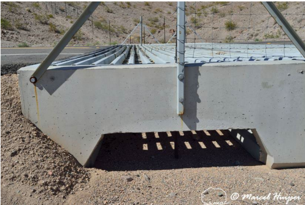
Figure 104. Combined drainage and escape for small animals under wildlife guard, Arizona, USA. The openings on the side allow for drainage under the culvert. The openings also allow invertebrates, amphibians, reptiles, small mammals and other species that may fall in between the metal bars to escape. For wildlife guards that have a fully enclosed pit with contiguous walls sometimes wooden planks or metal strips are attached, allowing animals to climb out of the pit.
