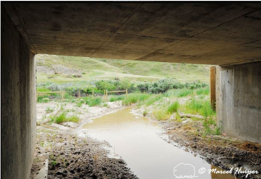
Figure 81. Bottomless culvert.
