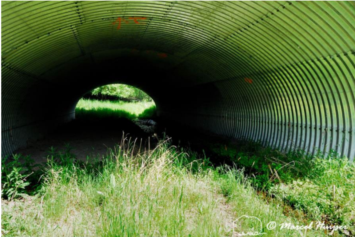
Figure 25. Multi-functional underpass for wildlife and water with soil and rocks that cover the bottom of the culvert, US Hwy 93, near St Ignatius, Flathead Indian Reservation, Montana, USA.
