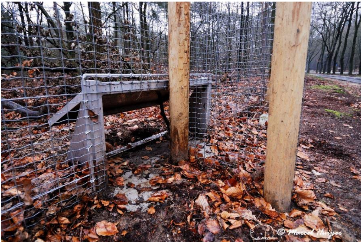
Figure 107. Escape gate for Eurasian badger ( Meles meles ) in wildlife fence Harderwijk, The Netherlands. Note that these types of gates are often left open because of debris which threatens their functioning.
