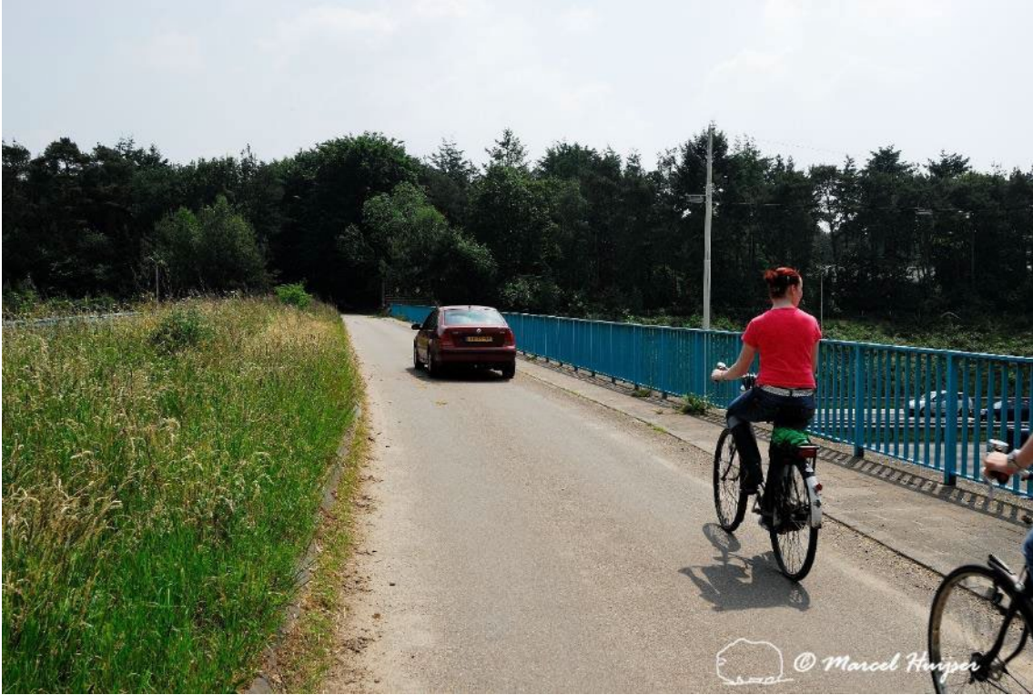
Figure 101. A bridge across the A28 motorway near Utrecht, The Netherlands. One of the lanes was later devoted to habitat for small animal species, including invertebrates.
