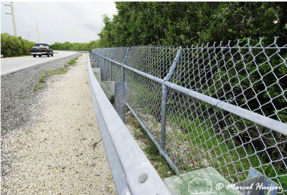
Figure 73. Fence with overhang for American crocodile ( Crocodylus acutus ), Key Largo, Florida, USA.
