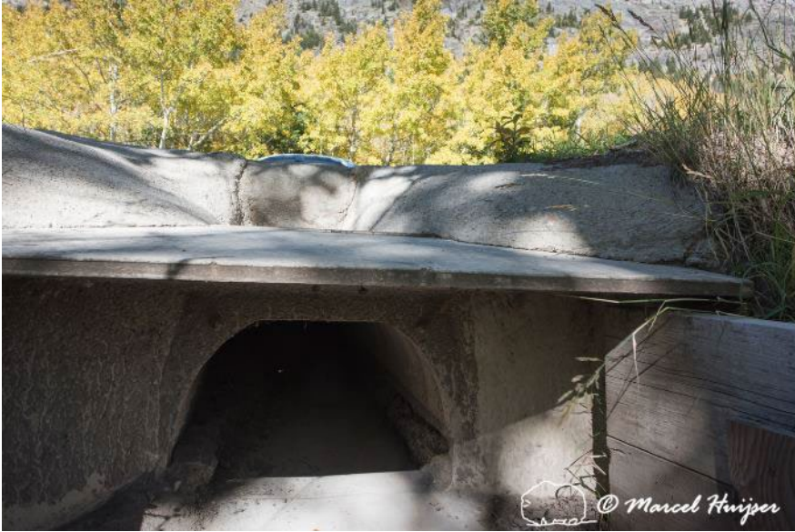
Figure 83. Culvert for long-toed salamander ( Ambystoma macrodactylum ), Waterton Lakes National Park, Alberta, Canada.
