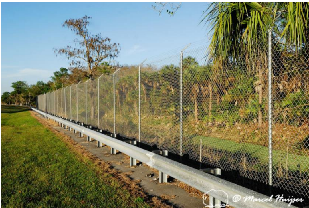
Figure 8. Fence for Florida panther ( Puma concolor coryi ), 10 ft tall, metal posts, chain-link fence material, and overhang, SR 29, Florida, USA).
