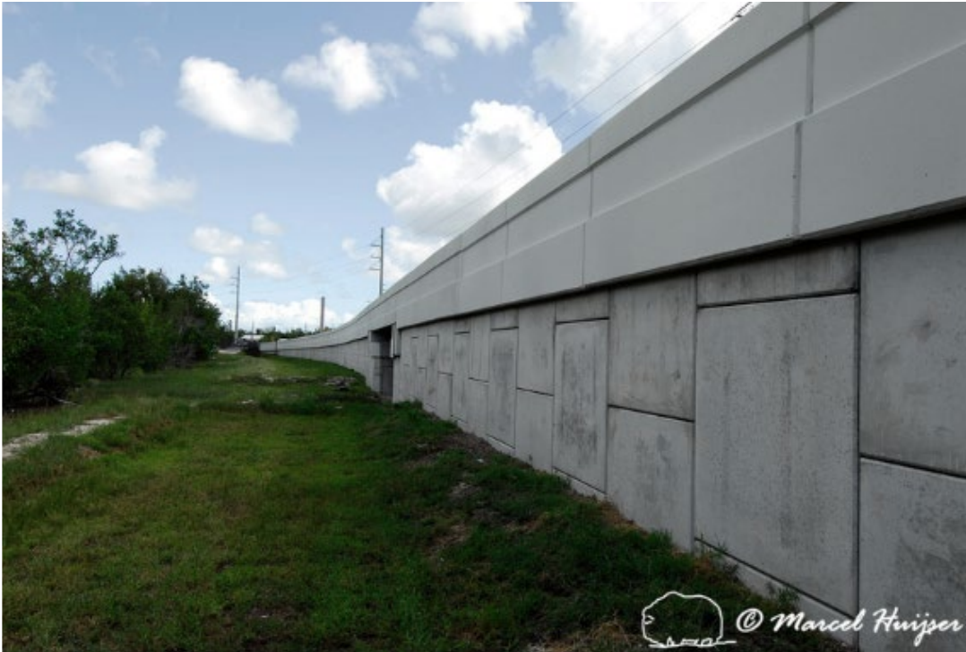
Figure 6. A barrier wall because of raised roadbed for wildlife underpass for Key deer (8 m wide, 3 m high), US Hwy 1, Big Pine Key, Florida, USA. A barrier wall can be considered if concerns for landscape aesthetics do not allow for a fence.
