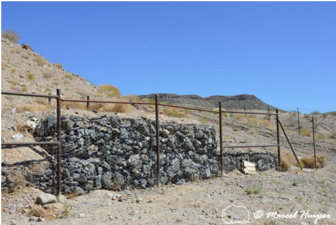
Figure 44. Wildlife jump-out or escape ramp with a rock wall and bar designed for desert bighorn sheep ( Ovis canadensis nelsoni ), US Hwy 93, Arizona, USA. The bar reduces the probability that bighorn sheep will jump up into the fenced road corridor while it does not decrease the probability that the bighorn sheep will jump down to the safe side of the fence. The sheep can crawl under the bar before jumping down.
