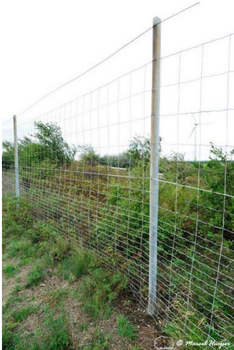
Figure 68. Mesh wire wildlife fence with metal poles on top of multifunctional overpass (wildlife, bicyclists, pedestrians; about 100 m wide), across A4 motorway, Parndorf, Austria. The overpass is designed for farmers, agricultural machinery, hunters and wildlife including roe deer ( Capreolus capreolus ) and European hare ( Lepus europaeus ). Mesh size is small towards the bottom.
