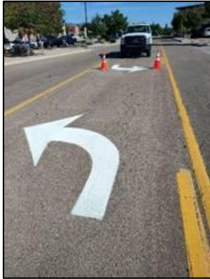
Roadway Striping on Central
