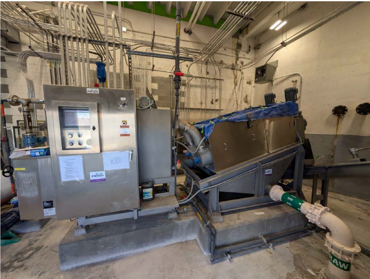
NEW BELT PRESS IN WHITE ROCK – SAME AS LOS ALAMOS REPLACEMENT
