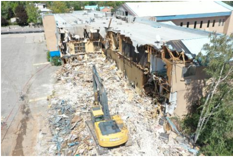
Hilltop House Demolition
