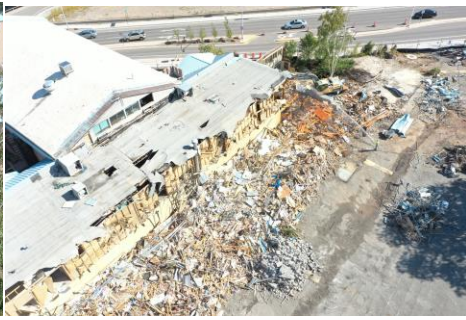
Hilltop House Demolition
