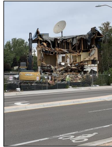
Hilltop House Demolition
