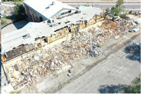
Hilltop House Demolition
