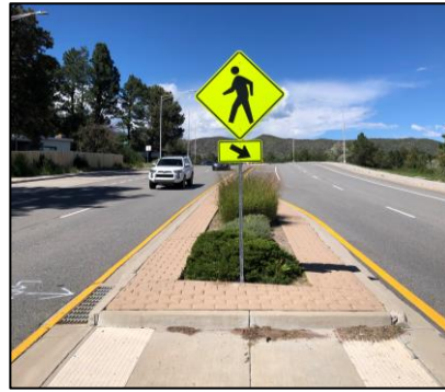
Installed new crosswalk signs
