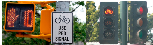
Figure 3.16: Options to enable leading bicycle interval at intersection, by either cyclists using the leading pedestrian light or having a separate bicycle light.
