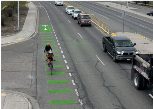
Green Bike Lane Installation
