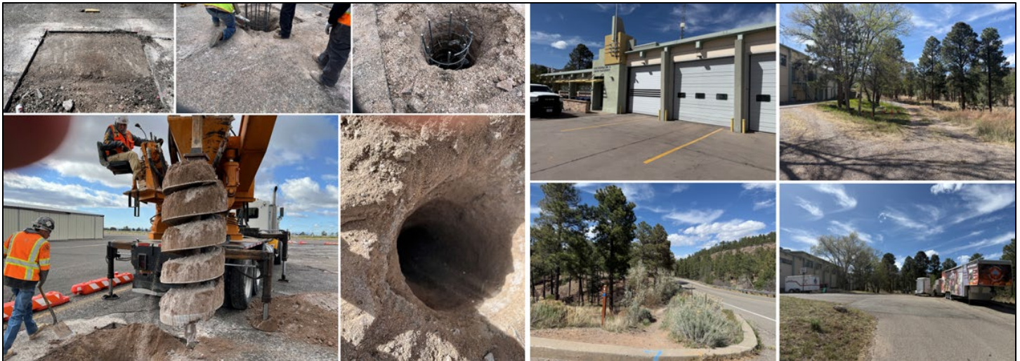
T-Hanger Concrete Pier Drilling
