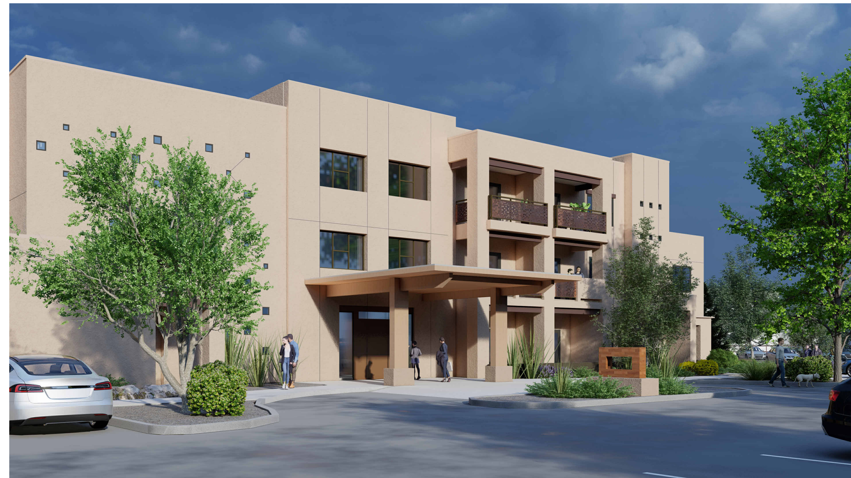
NOTE: IMAGE IS CONCEPTUAL IN NATURE AND MAY NOT REFLECT THE REQUIREMENTS OF THESE PLANS
