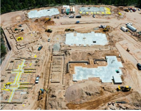
Photo from July 2022 showing poured foundation slab as well as foundation forms and retention wall in place
