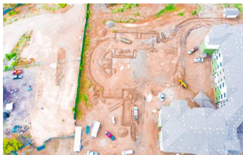
Aerial showing grading and form setting for curbs.
