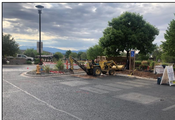
Construction is underway at White Rock Visitor Center to improve water pressure to the building. Trenches are being hand-dug to avoid striking underground utilities.
