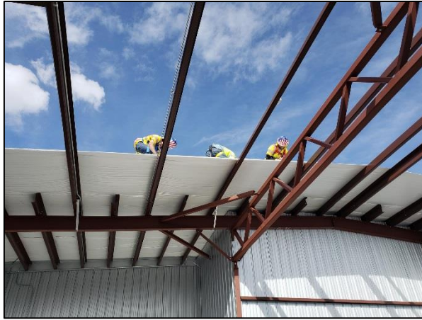
Crews install roofing on the new hanger structure
