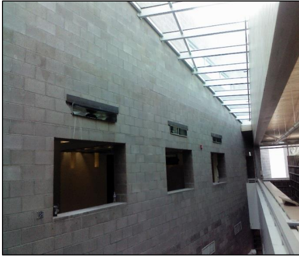
New return air penetration (smaller holes)
