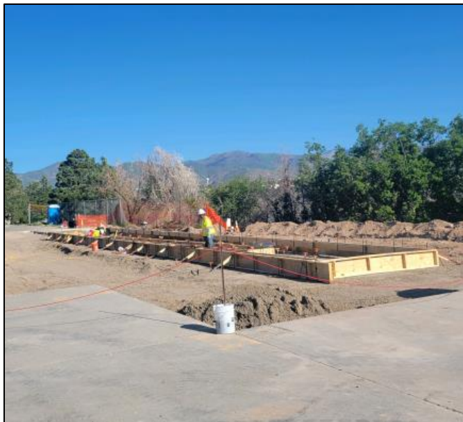
Airport Fuel Farm Project
