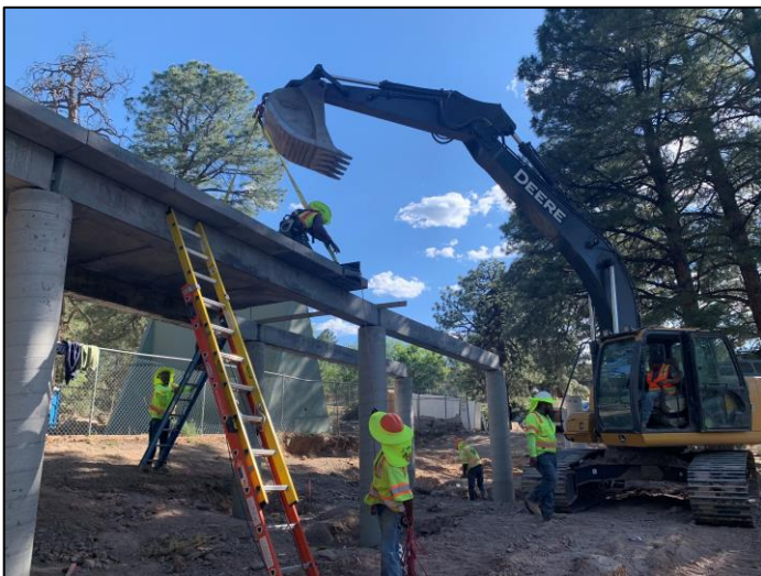
Urban Trail –installation of boardwalk
