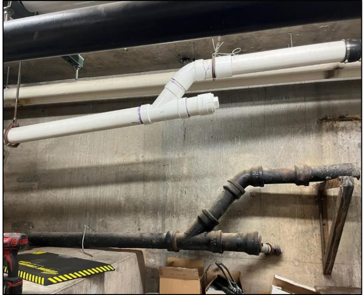
Facilities repaired a sewer drain line at Fuller Lodge
