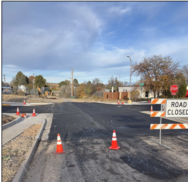
Streets crews excavated, prepared and laid asphalt and repaired a culvert that eroded at the intersection of Aragon and Cheryl Avenues.
