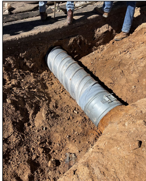
Streets crews excavated, prepared and laid asphalt and repaired a culvert that eroded at the intersection of Aragon and Cheryl Avenues.
