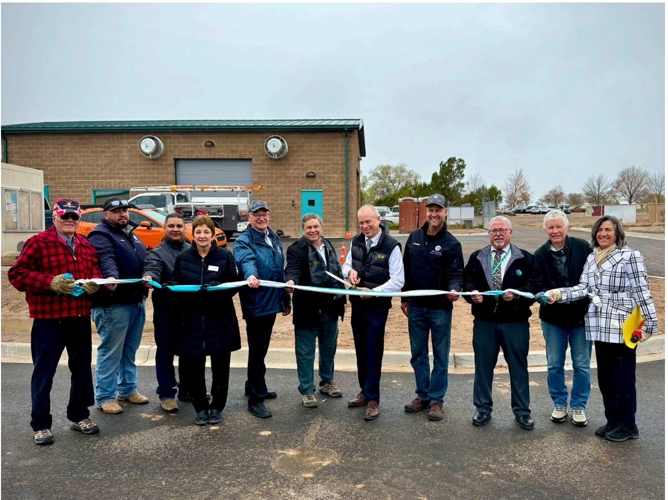
Though it turned out to be a cold and blustery day with a little bit of snow in the air, November 6 was a day to celebrate at the ribbon cutting for the White Rock Water Resource Reclamation Facility. Pictured above are BPU Chair Robert Gibson, WWTP Superintendent Joshua Silva, Senior Engineer James Martinez, County Council Chair Denise Derkacs, Utilities Manager Philo Shelton, County Councilor David Reagor, NMED Secretary James Kenney, Deputy Utility Manager Clay Moseley, NMED Deputy Secretary John Rhoderick, County Councilor Theresa Cull and Deputy County Manager Linda Matteson
