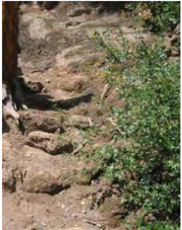
Improve stairs near 34th Street.
