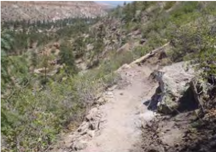
Monitor condition of switchbacks throughout the trail.
