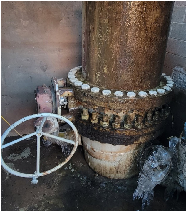
Left: Ice coats equipment due to the leaking valve assembly on Abiquiu's penstock vent valve. Right: A blind flange was installed on the valve to remedy the leak.
