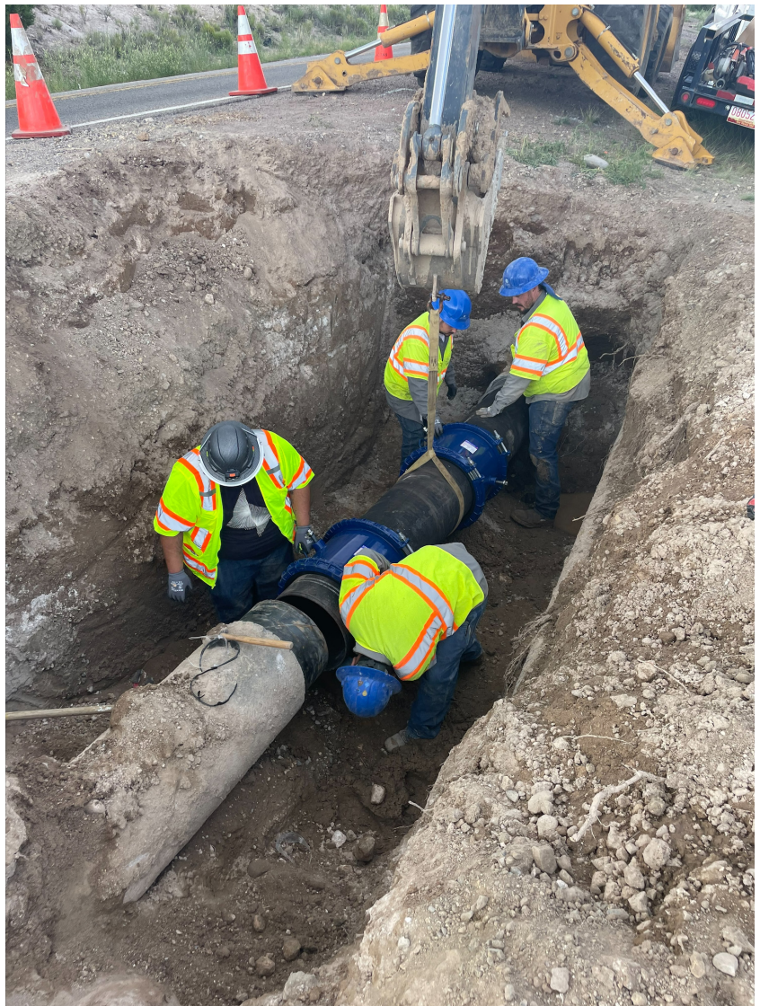
Water Production crews repaired the transmission pipeline along NM-4 just weeks before its replacement project began.
