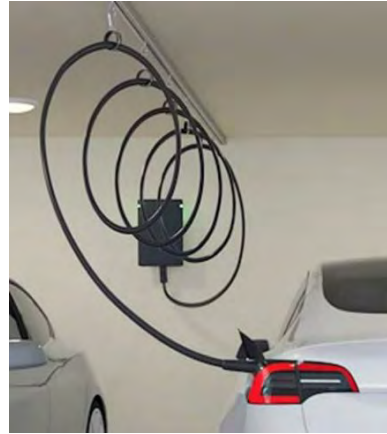
Figure 2-5: Examples of cable management for overhead dispensers
