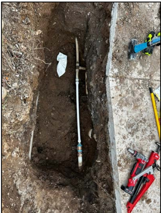
Leaking water pipe repaired at Nature Center.
