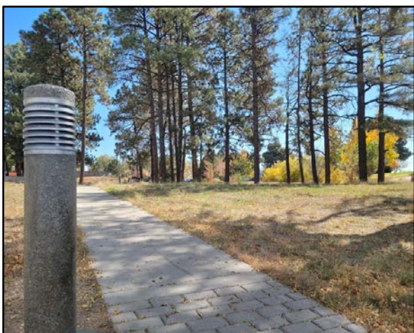
Bollards replaced at Mesa Public Library.
