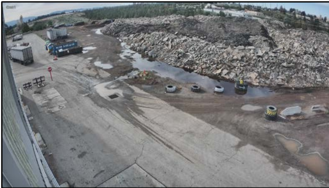
Concrete at Eco Station Before
