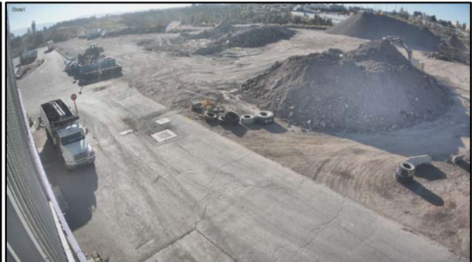
Concrete at Eco Station After
