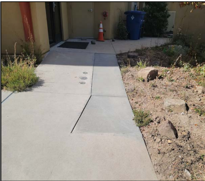
Concrete replaced over repaired water pipe at Nature Center.
