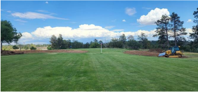
New fairway bunkers on Hole
