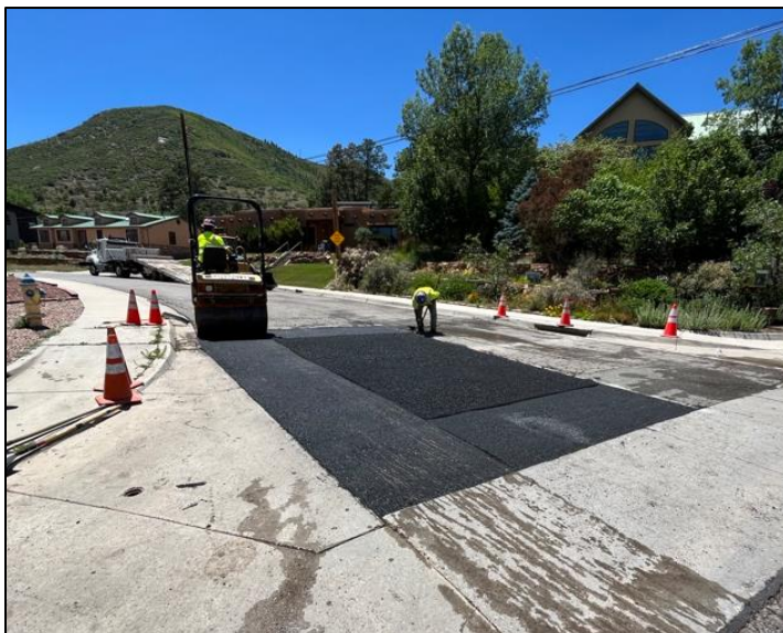
Crews patching in preparation for the crack seal project.
