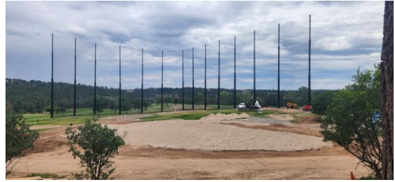
Large Pole Netting Complete
