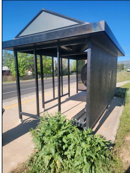
Crews repaired the bus structure near the middle school.
